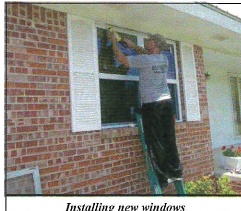
Installing new windows
