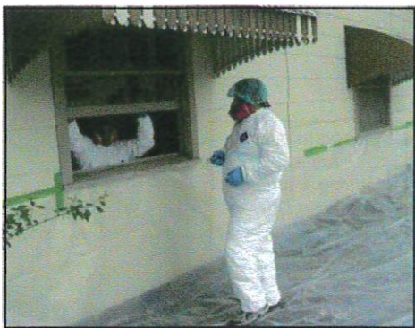
Removing lead-base paint from a client's home
