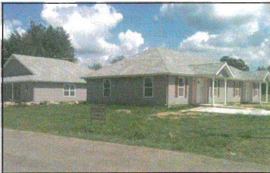
New Duplexes under construction in Jay
