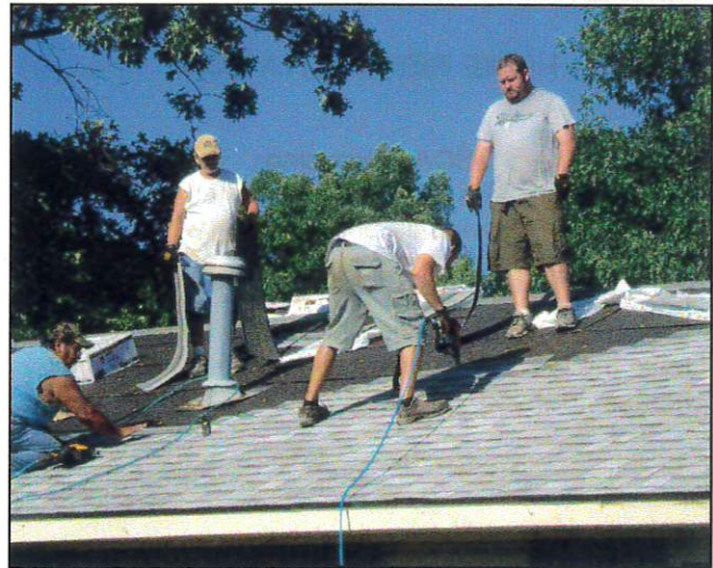
Installing a cool roof
