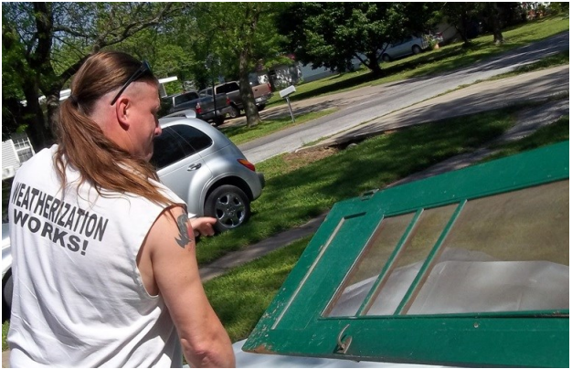
Doors and Windows are repaired or replaced
