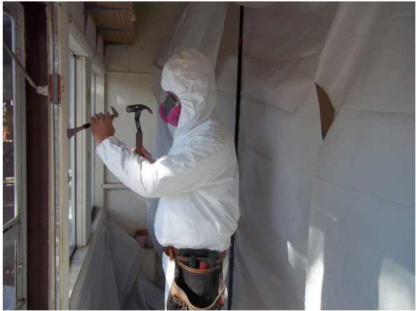
Tyvek suits are worn during safe work practices for windows with lead base paint
