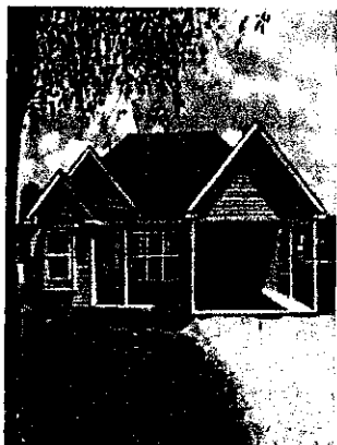
638 14" St. lay, OK Built 2015
