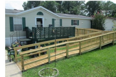
Ramps, Roofing, Electrical, Siding, flooring, bathrooms, kitchen etc.
