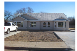
Tahlequah New Construction Rental Housing
